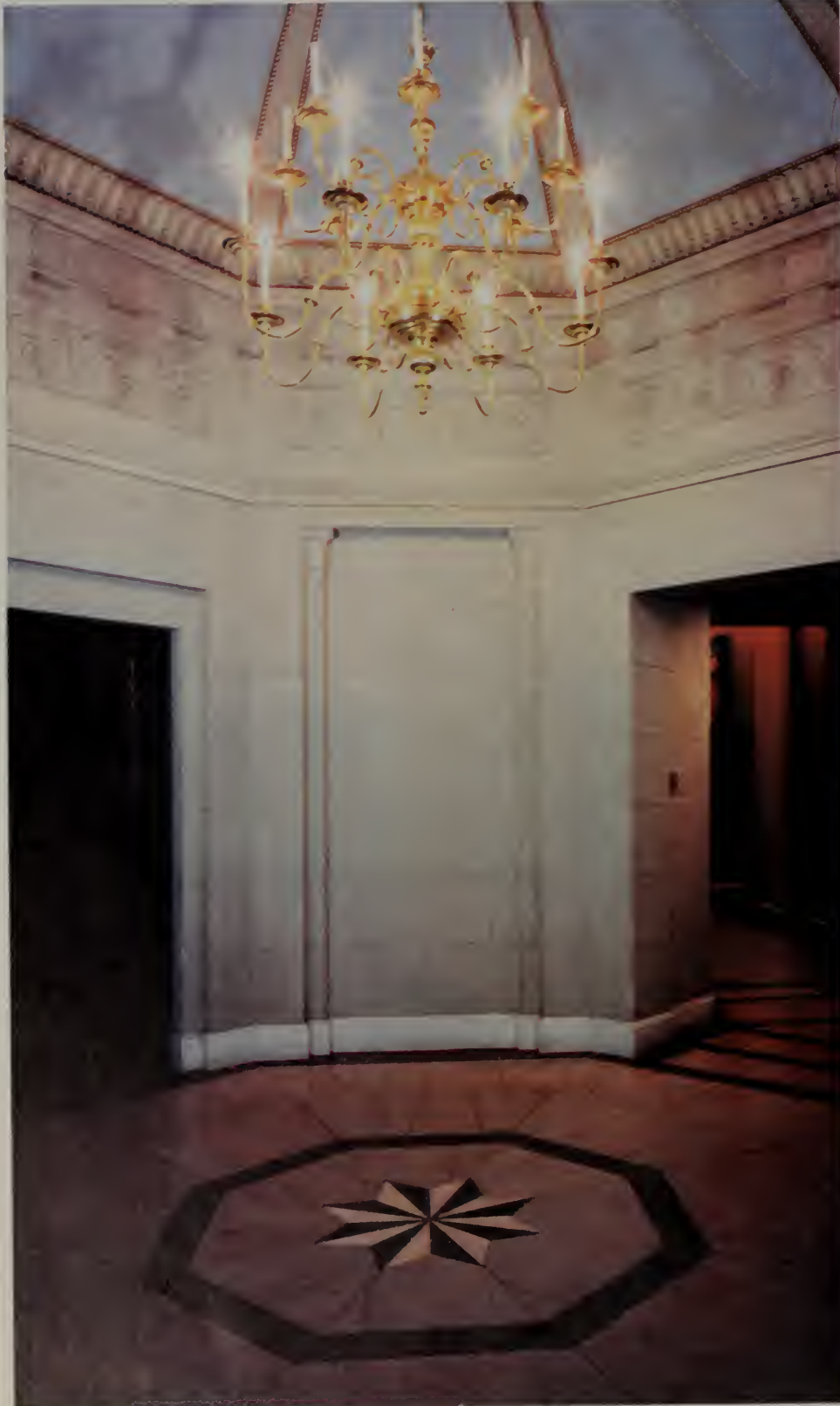
Second floor passageway after modification. Caen stone walls, octagonal marble floor, ornamental plaster ceiling and appropriate chandelier embellish the space.
